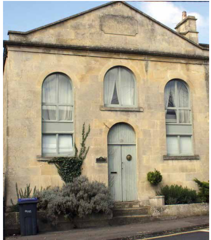
Sladesbrook Primitive Methodist Chapel became a Temperance Hall towards the end of the 19th century
