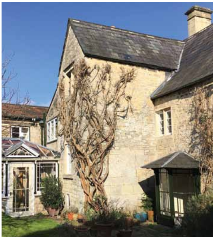
◀ Back of the house showing part of the rear wing and conservatory, the staircase tower with the possibly re-used Roman stones and the French window in a bay leading off the 'hall'
