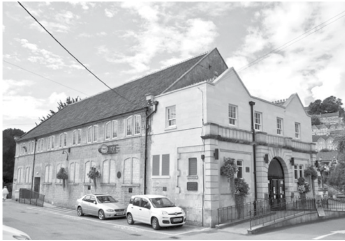
St Margaret's Hall today – the old projection box was sited immediately above the foyer
